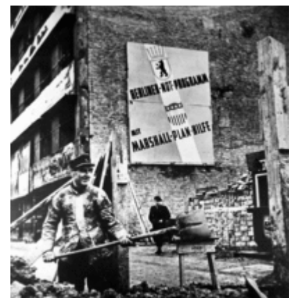
Construction in West Berlin under Marshall Plan aid
