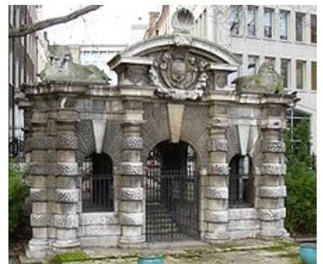
The Italianate entry to York House , built around 1626 in Strand , the year of Bacon's death
